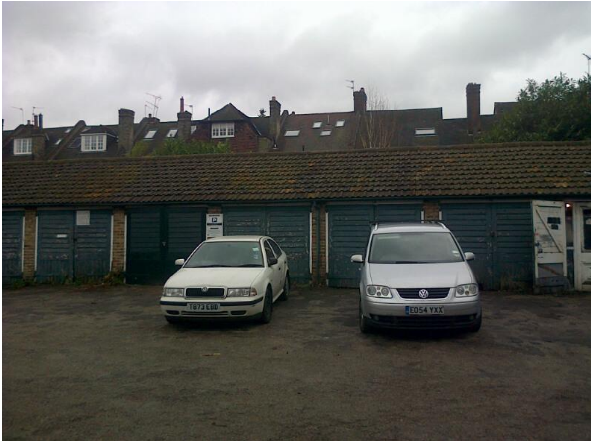
View of garages and rear of Cranmore Way properties
