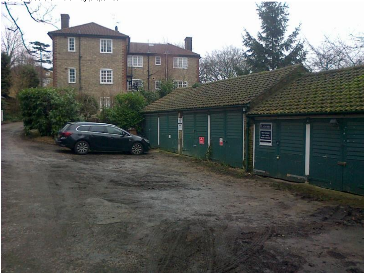
View of existing garages adjacent to the entrance
