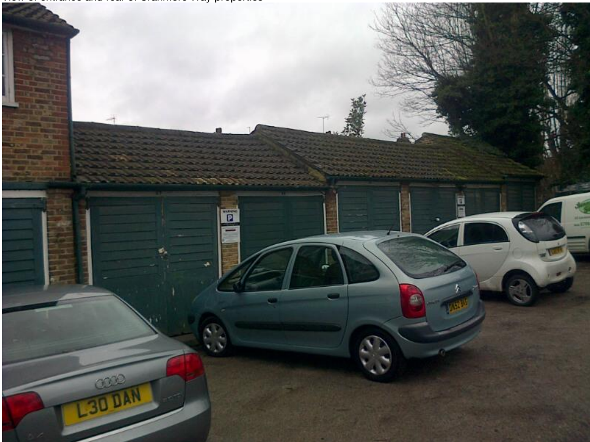
View of garages and cottage
