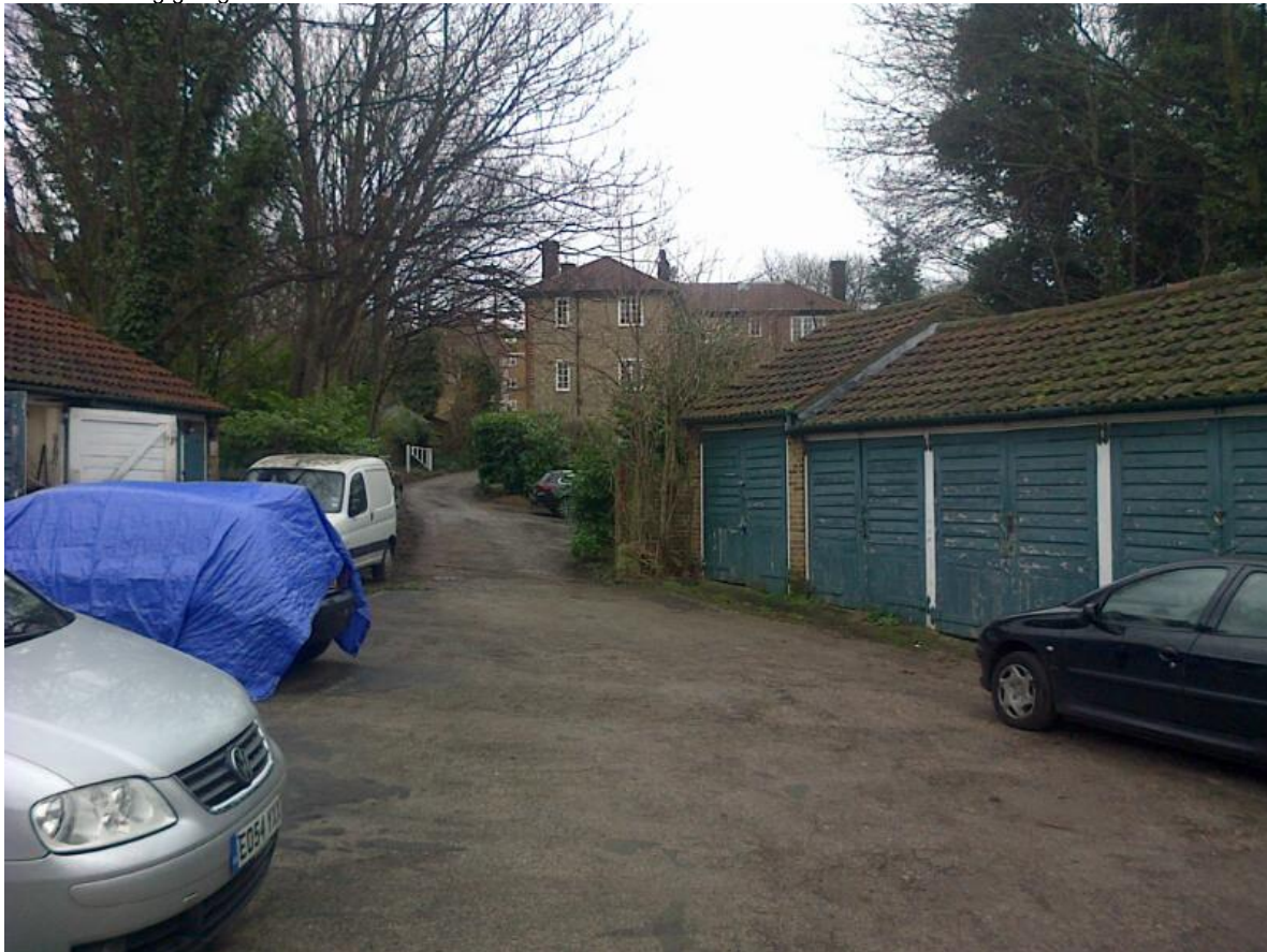
View of existing garages towards entrance 2
