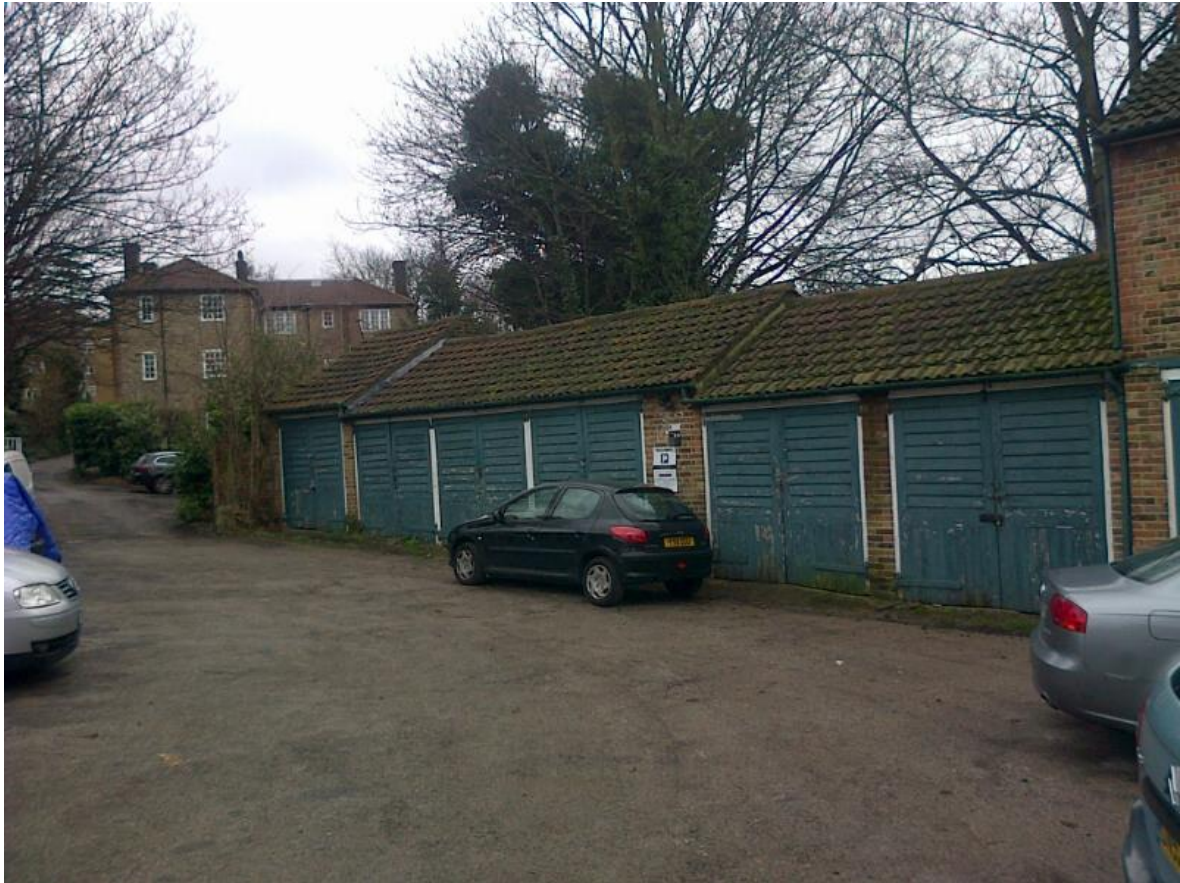
View of existing garages towards entrance 1
